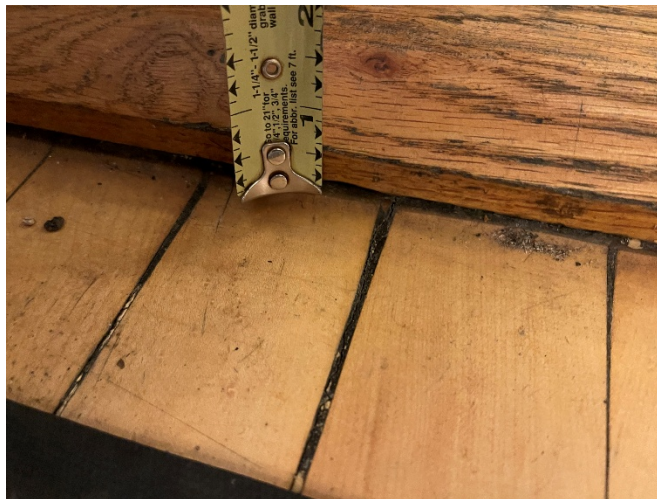
Figure 6 - Photo of threshold vertical edge being measured
