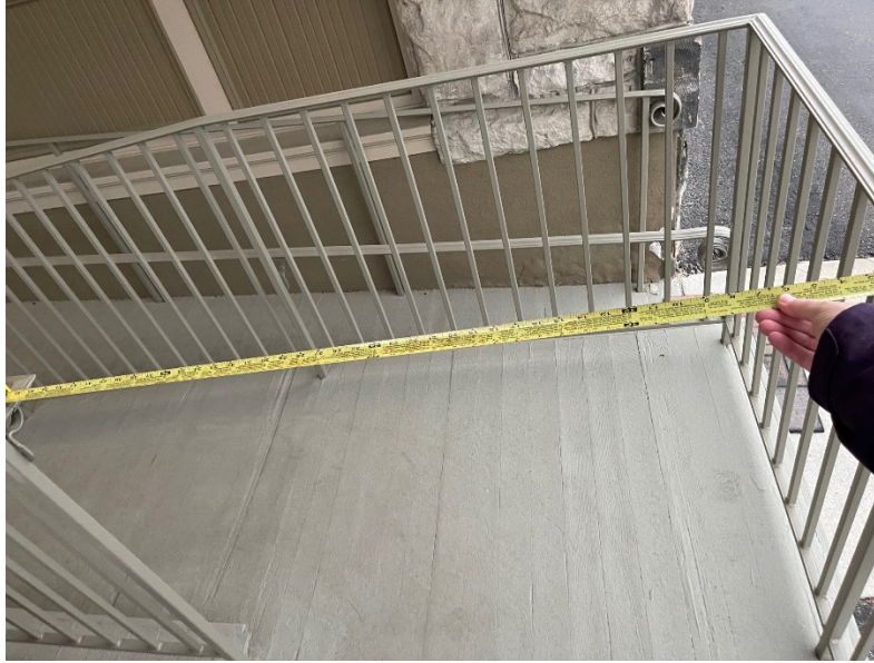
Figure 4 - Photo of ramp landing being measured
